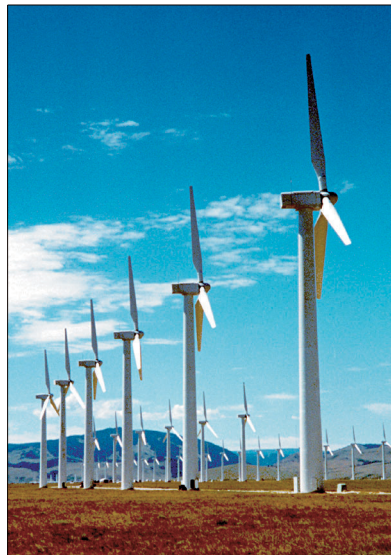
Foote Creek Rim Wind Farm
