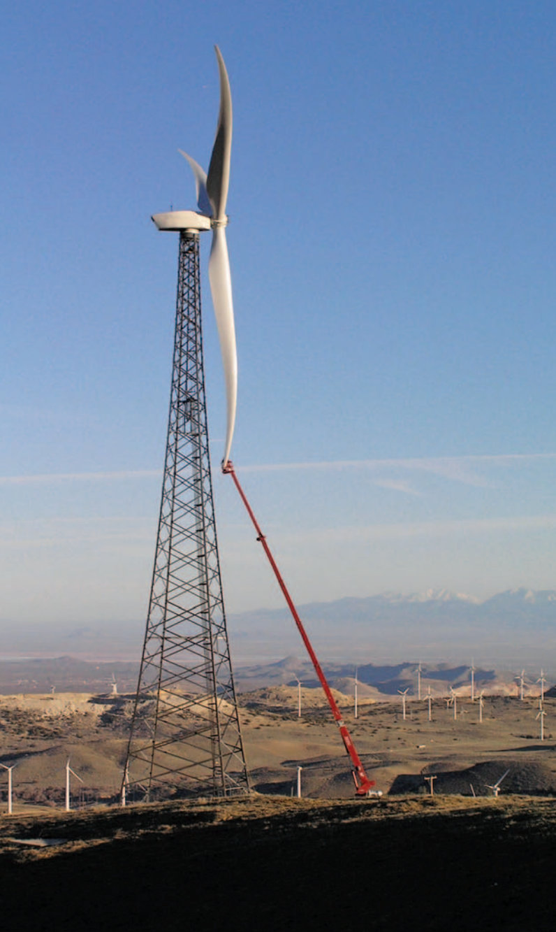
The DOE Wind Program worked with Knight & Carver to develop an innovative wind turbine blade that the company expects to increase energy capture by 5% to 9%. The most distinctive feature of the Sweep Twist Adaptive Rotor (STAR) blade is its gently curved tip.
