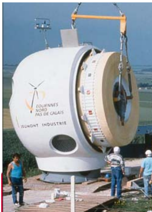
Figure 4-14. Installation of Jeumont J-48 direct-drive turbine with PM axial flux generator.
