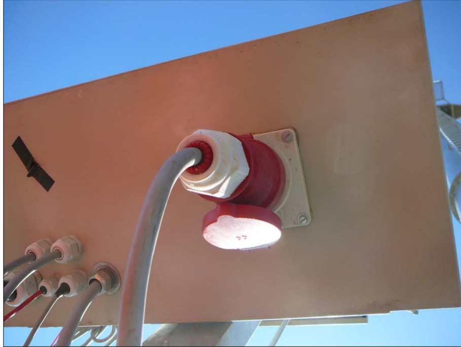
Figure 17. Power cable termination at controller
