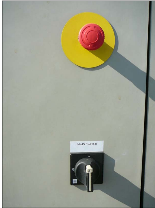
Figure 15. Gaia-Wind 11 kW emergency-stop button and main switch
