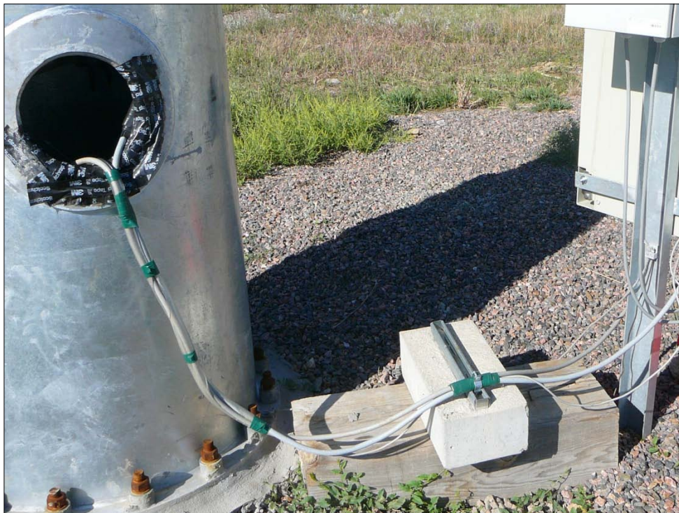
Figure 16. Power and instrumentation cables from turbine to controller
