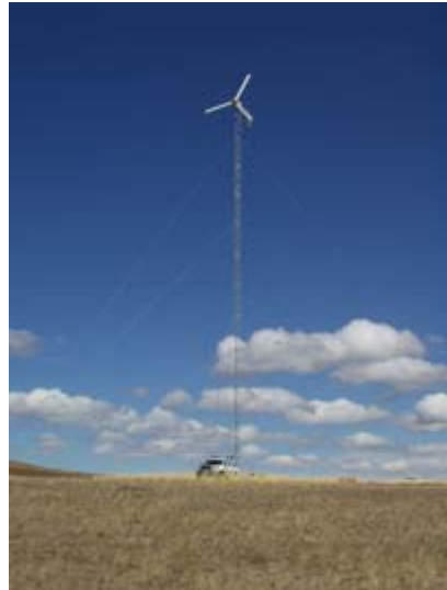
Figure 4: Turbine installed in field behind Bassetti ranch. Source: NWSEED
