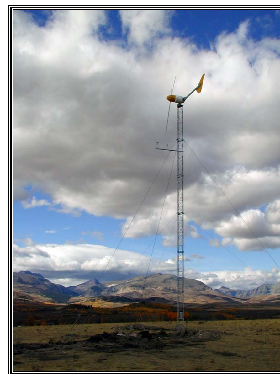
Tower type/height: 18m standard guyed. Commission date February 20, 2004. Host site: Doug Nelson.
