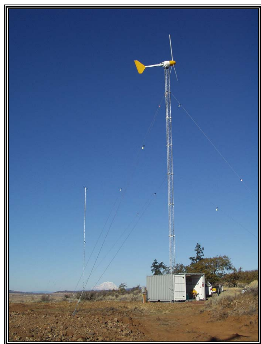
Tower type/height: 24m standard guyed. Commission date October 31, 2003. Host site: Ed Kennell.
