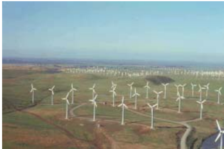
Figure 20. NREL photo PIX00052 with a pale blue sky and brown and green at ground level. Photo credit: Warren Gretz.
