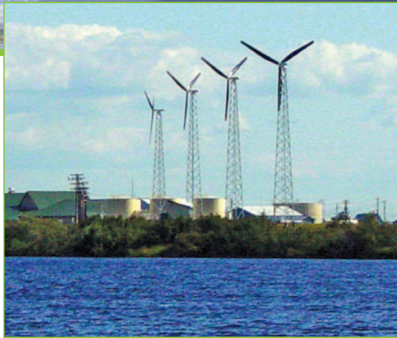
Alaska Village Electric Cooperative Inc. installed four 50-kW turbines in Selawik, which is located 3 miles north of the Arctic Circle. Alaska Village Electric Cooperative/PIX13055.
