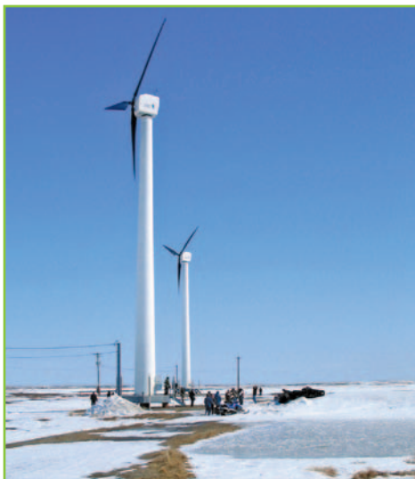
Kasigluk turbines. Ian Baring-Gould/PIX16096.
