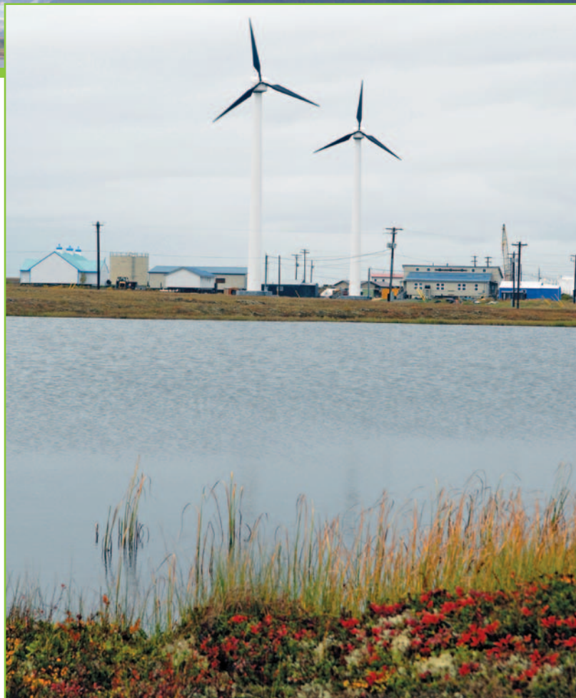
Wind turbines at the Kasigluk project. Northern Power Systems/PIX15391.
