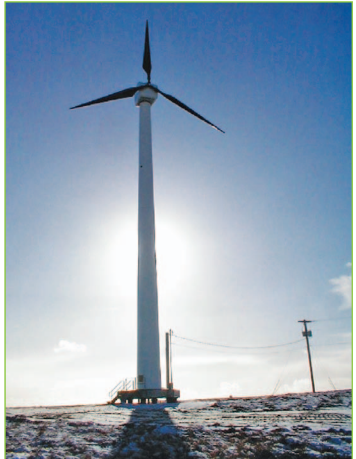
Three 100-kW Northern Power Systems Northwind 100 turbines were installed as part of a power system upgrade to serve the community of Toksook Bay, Alaska. Photo credit: Northern Power Systems/ PIX14406 (top), PIX14401 (bottom left), PIX14405 (bottom right).
