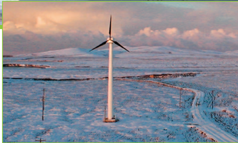
Three 100-kW Northern Power Systems Northwind 100 turbines were installed as part of a power system upgrade to serve the community of Toksook Bay, Alaska. Photo credit: Northern Power Systems/ PIX14406 (top), PIX14401 (bottom left), PIX14405 (bottom right).
