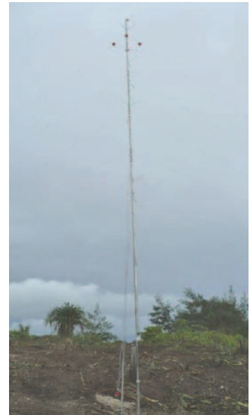
A 60-m met tower was installed on the western ridge of a Navy installation on Guam. Credit: DNV Global Concepts Inc., PIX16289.
