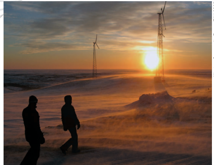
Western Community Energy/PIX16305
